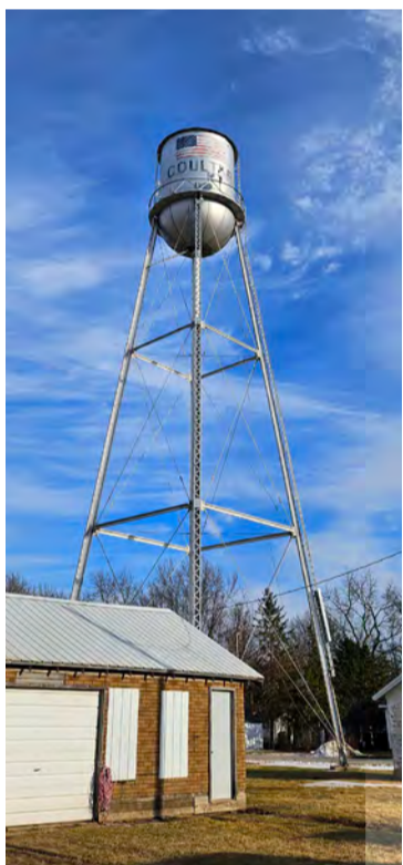
The Coulter water tower makes sure the Coulter Fire Department gets the water pressure it needs to save property and lives in Coulter and Hamilton and Morgan townships.
